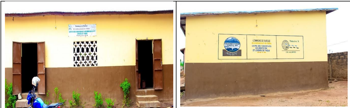
6. Through the project of creation of a recreative space inside the main group of schools, (i)- a hall of 100 m2 has been built to serve as both conference room and library for the pupils.
